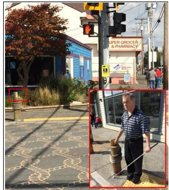
A good example of a raised intersection with accessible pedestrian signals and attention TWSIs. The top of the bollard is cut to indicate the direction of crossing.
